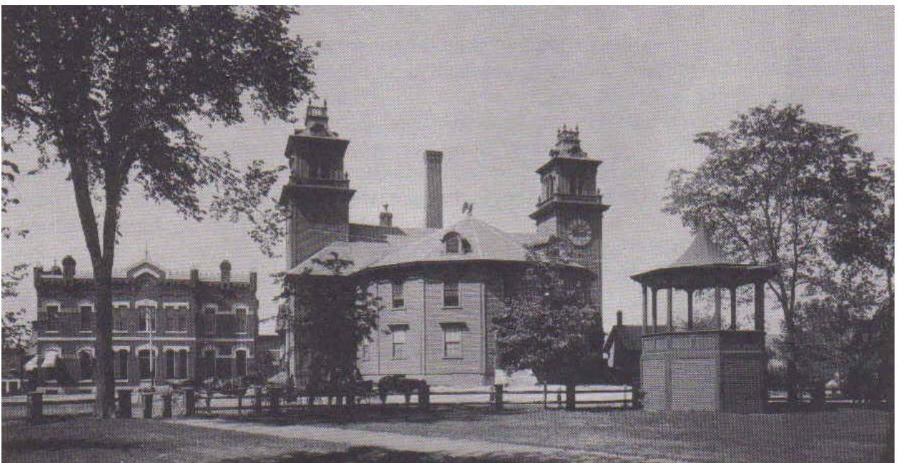
Claremont's old two-towered Town hall, demolished to make way for the Opera House.
