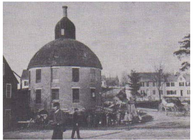
Round House and Elm Street – built in 1859 by Simeon Ide to house his printing presses and other machinery.
